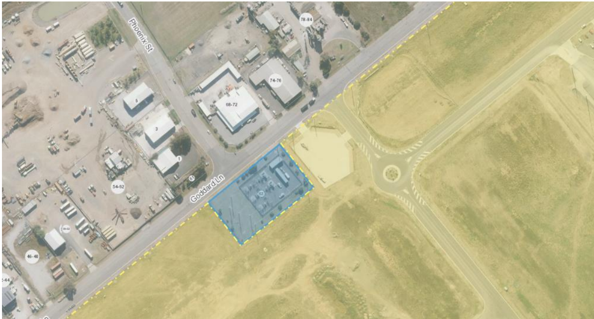
Figure 1 – Goddard Lane zone substation (blue) adjacent to TGGP (yellow)
