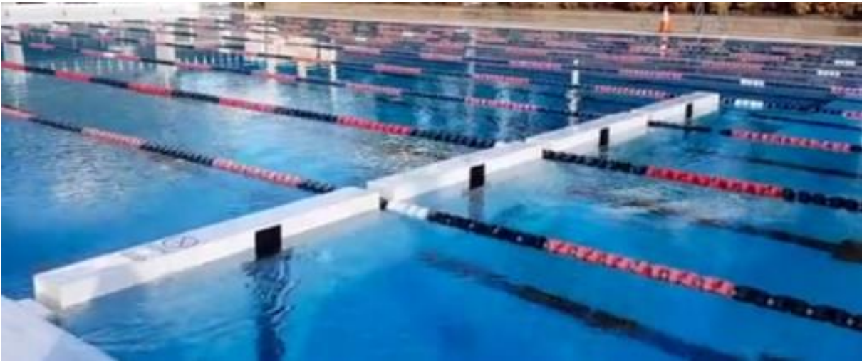
Figure 3 – Two-part swim wall with one part in use (left) and the other part stored on the floor of the pool (right).
