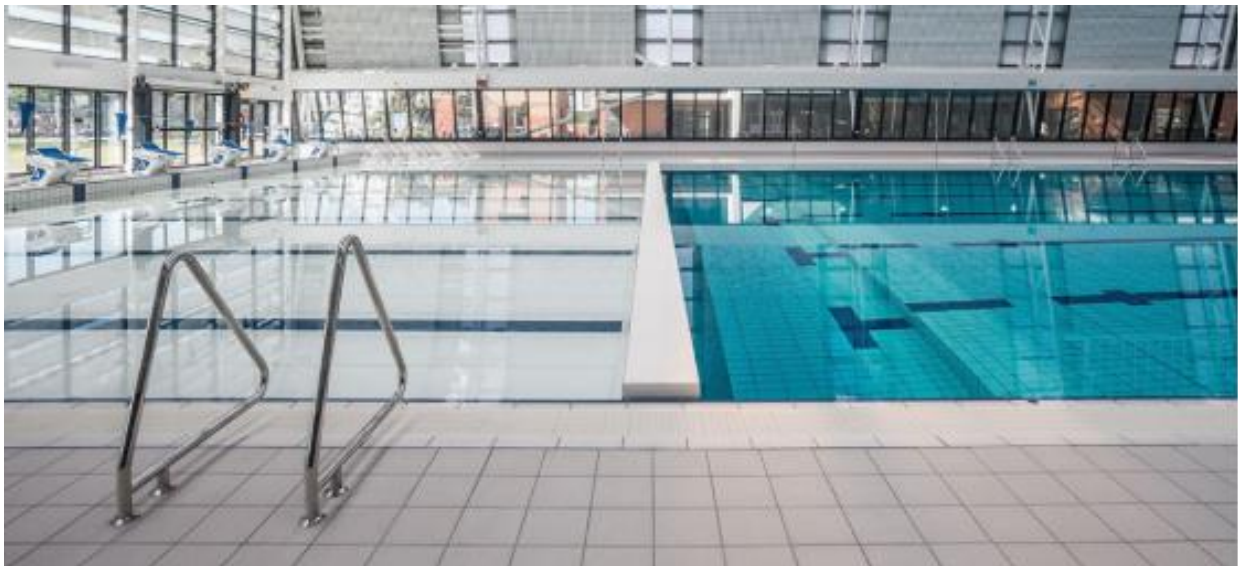
Figure 2 – Moveable floor (left) with swim wall in use (middle) with the floor rebate visible for when the wall is not in use (right).
